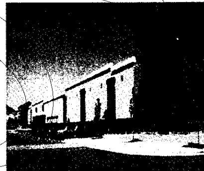
Figure 18.12-11.4: Side or rear walls that face walkways may include false windows and door openings defined by frames, sills, and lintels, or similarly proportioned modulations of the wall.
